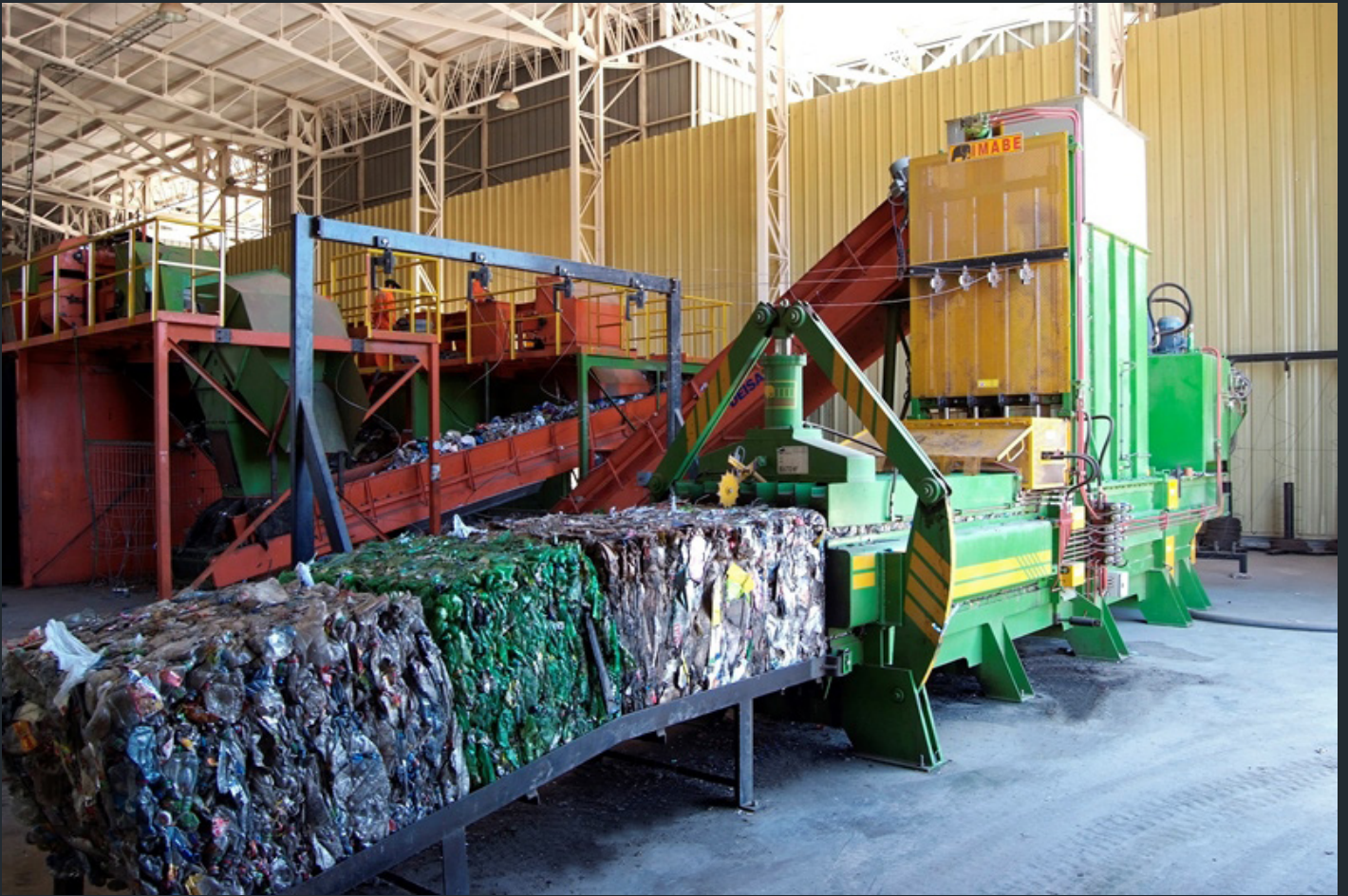
Recycling Plant. Source: Green Tracker
