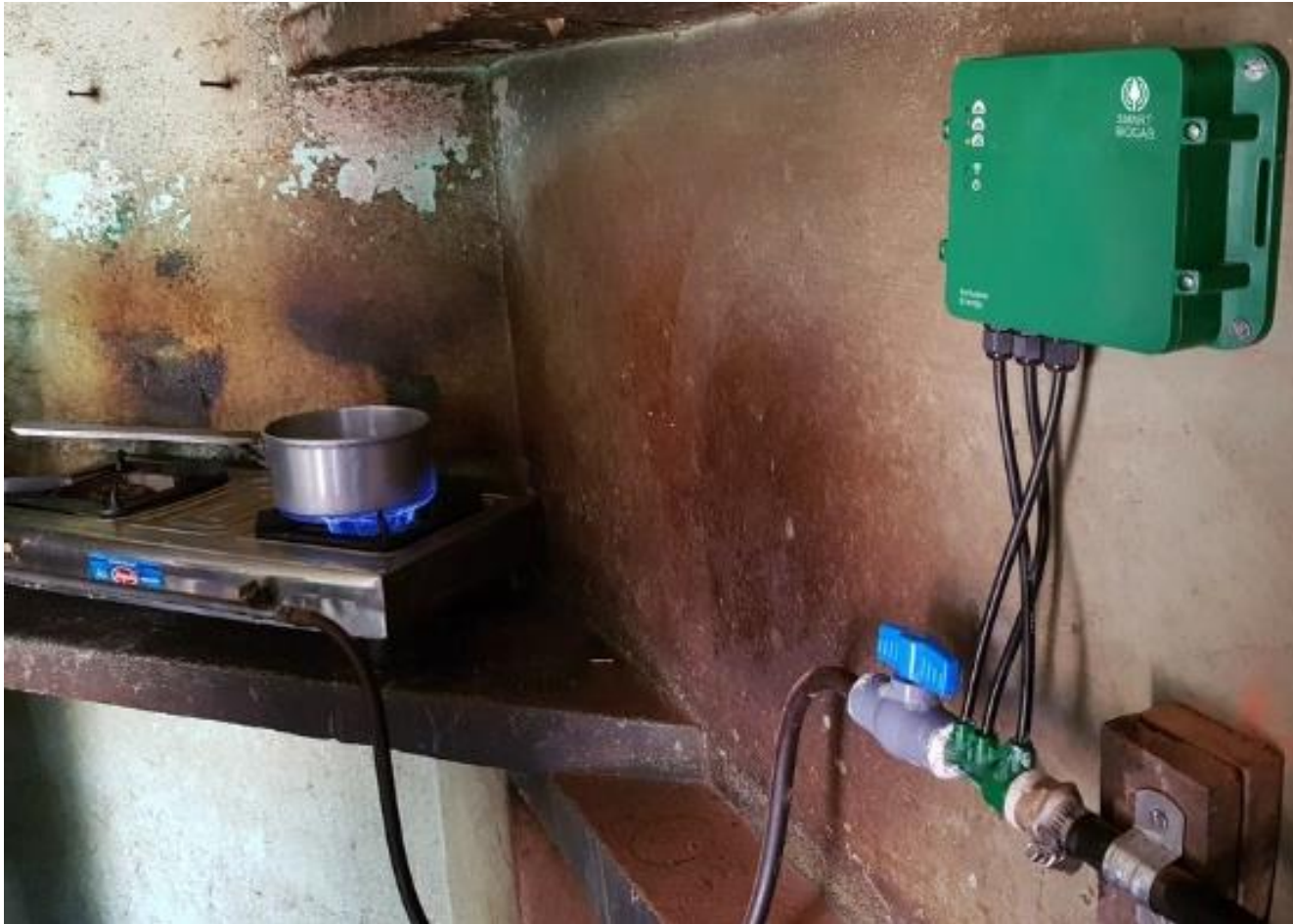
Source: Inclusive Energy Ltd
